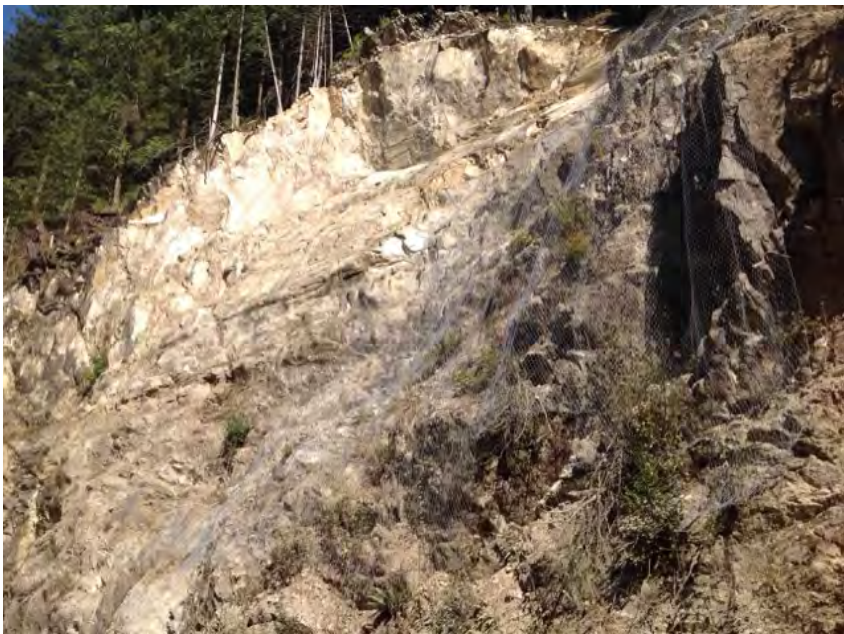
left bank cut slope
