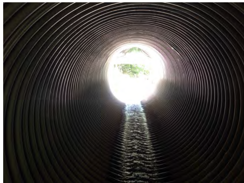
looking through culvert
