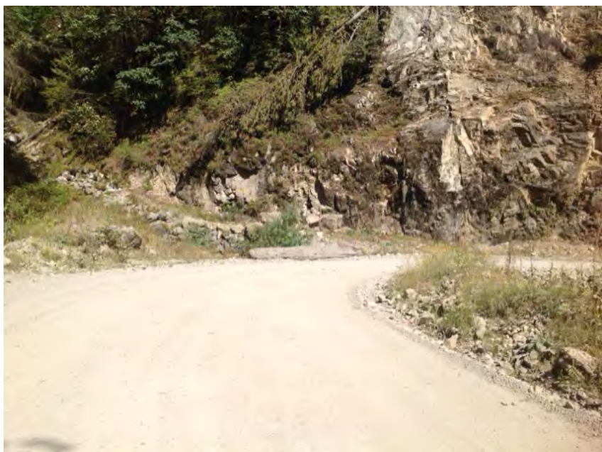
Approach from Right Bank when facing downstream
